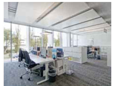
Multifunction exposed ceiling in an office
