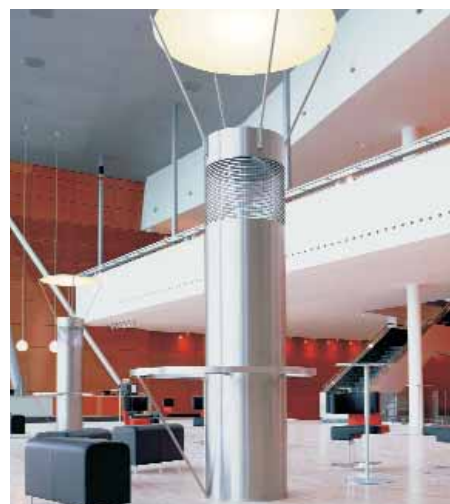
Luxor Theater, Rotterdam / NL Verdringingsrooster, Type Q-Z (blz. 16, 4.2.1.)
