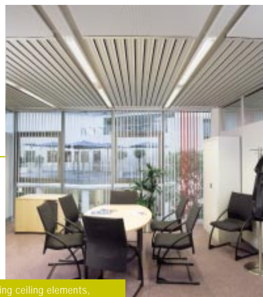
Metal lengthwise ceiling with acoustic coating (micropore)
