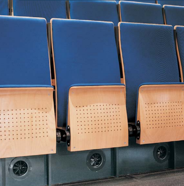
Step twist outlet, type DS-DD, in a lecture hall at the University of Amsterdam / NL
