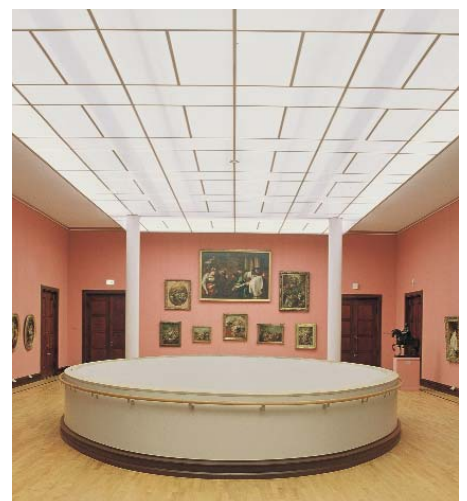
Plinth displacement outlets at 'Kunsthalle Bremen' / D
