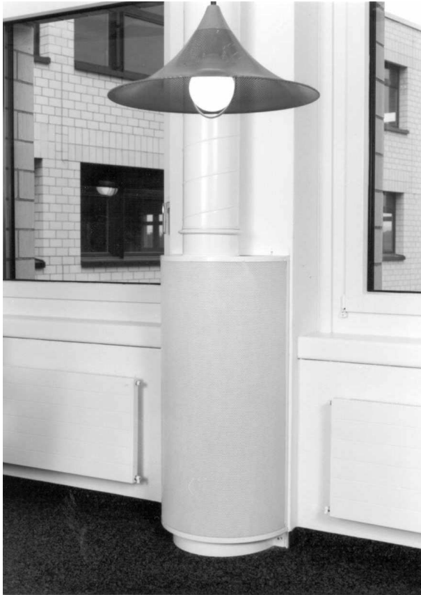
Semi-circular placed in front of a pillar
