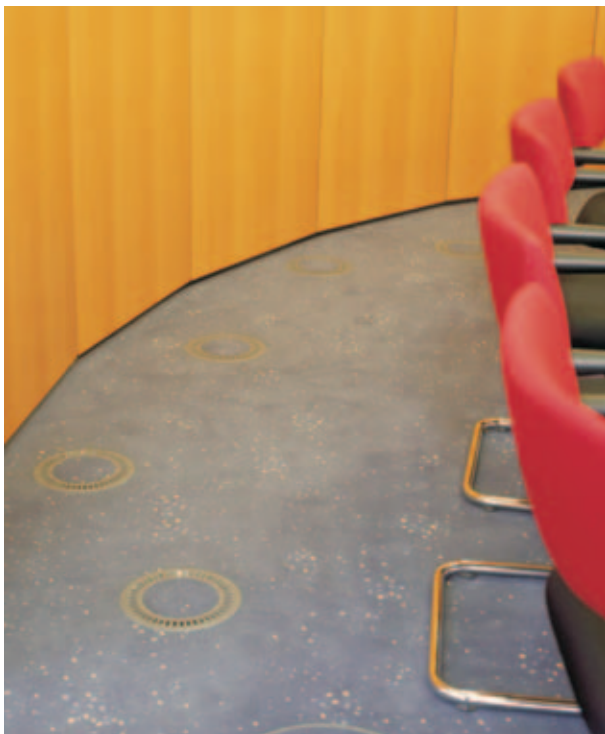
Fig. 3: Floor displacement outlet in a meeting room
