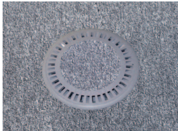
Fig. 2: Floor displacement outlet in a raised floor
