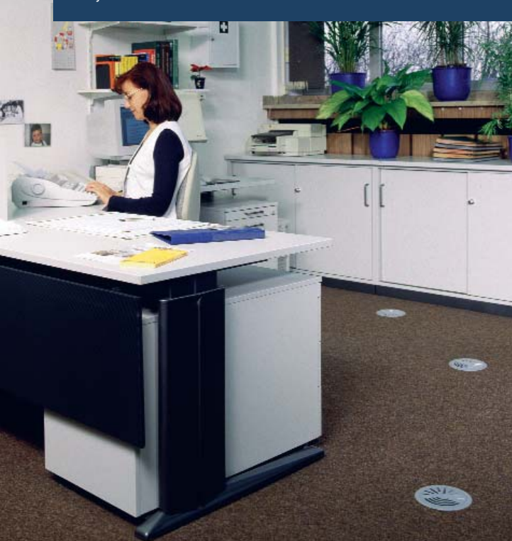
Rotary floor twist outlet in an office
