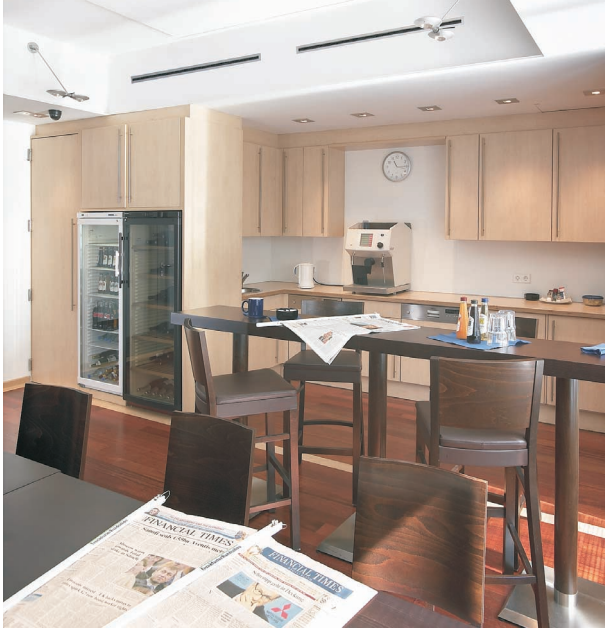
Fig. 3: Wall slot diffuser in the recreation room of an office building
