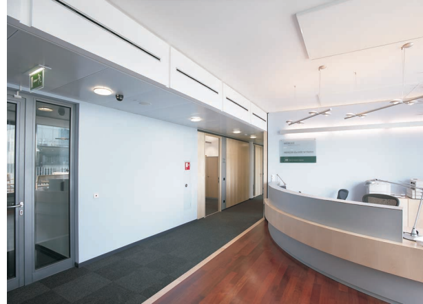
Fig. 4: Wall slot diffuser in the entrance area of an office building
