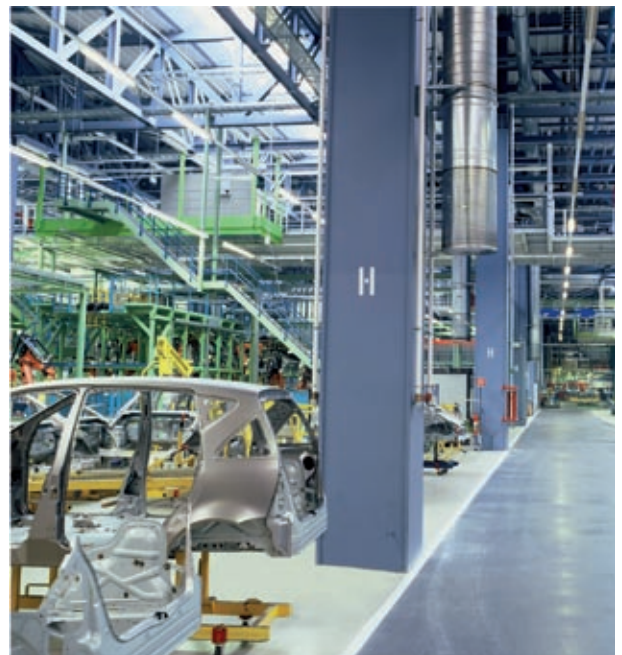
Fig. 13: Circular displacement outlets in car manufacturing halls
