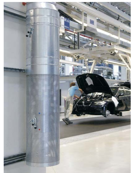
Circular displacement outlet, type VA-ZD, at 'BMW AG', Leipzig / D (Photographer: Martin Klindtworth)
