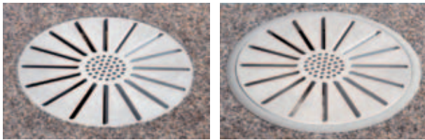
Figure 1: Floor displacement outlet in a floor tile
