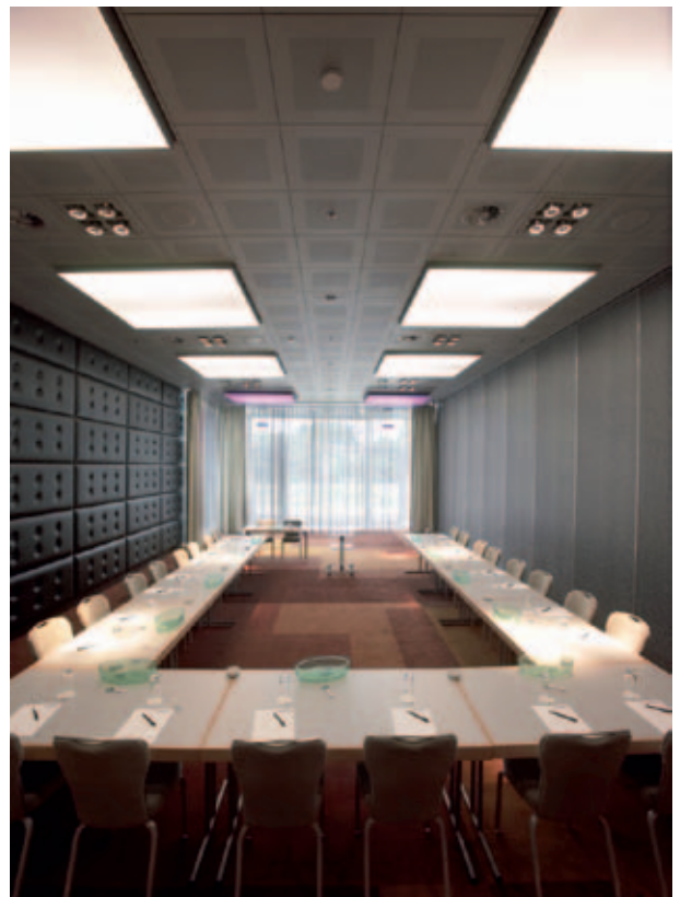
Fig. 5: Adjustable radial outlet in the meeting room of a hotel
