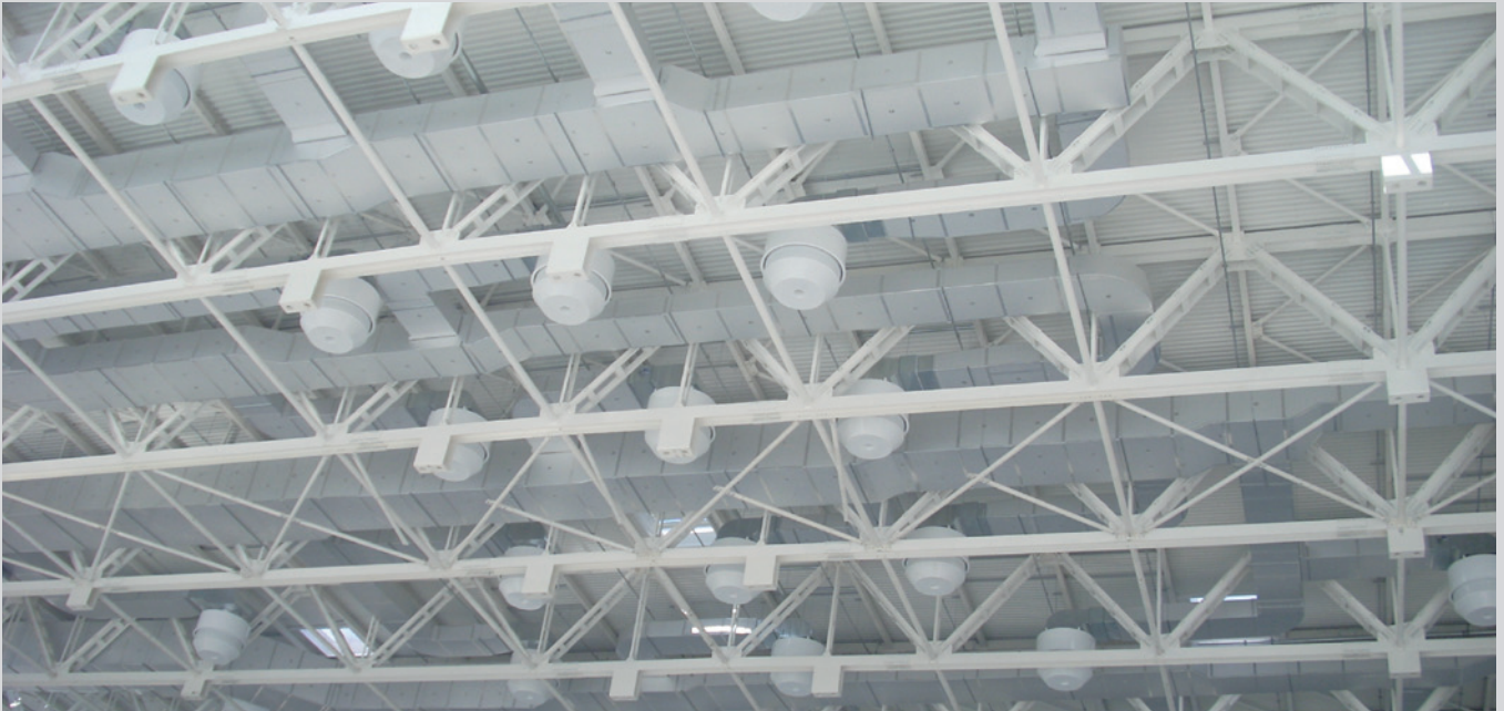
14 Conical displacement outlets in an aircraft painting hangar
