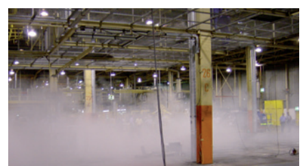
4 Stratified ventilation with air outlets positioned on the floor
