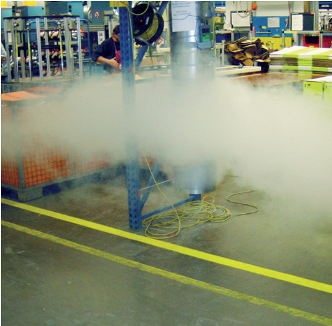
8 Displacement ventilation (stratified ventilation) while cooling
