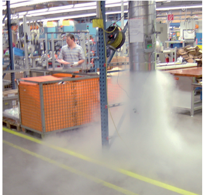
9 Displacement ventilation (stratified ventilation) while heating
