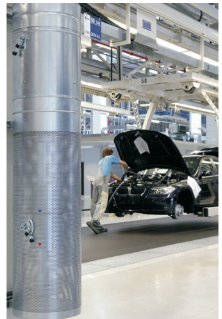
10 Air outlet with manual adjustment for stratified ventilation
