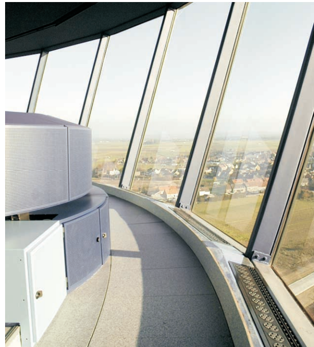
Fig. 5: Parapet outlet in an airport tower (Belgocontrol in Brussels)
